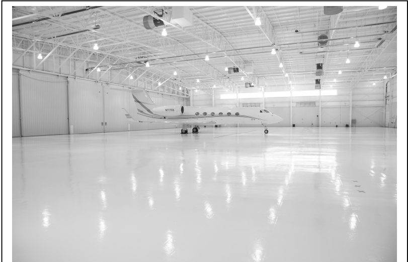
Open Web Frames – General Industries, Charleroi, Pennsylvania Photo courtesy of Don Ivill
