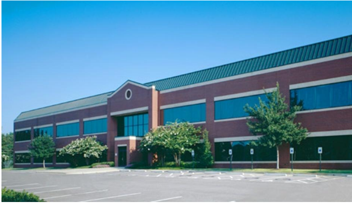
Varco Pruden Buildings Memphis, Tennessee
