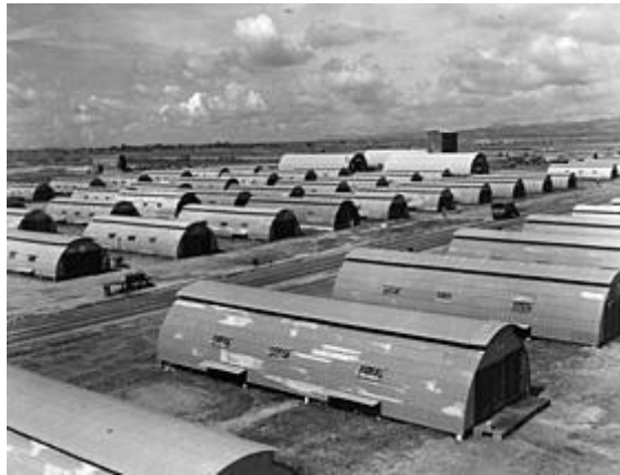
Stran Steel Quonset Huts - 1944 http://www.quonsethuts.org/huts/index.htm
