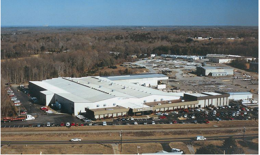
Varco Pruden Buildings – Kernersville, North Carolina ca. 2007
