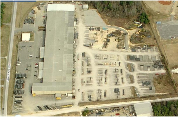
Varco Pruden – Rainsville, Alabama ca. 2007
