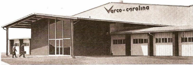
Varco-carolina Facility From Varco-Sparks Newsletter June 1967
