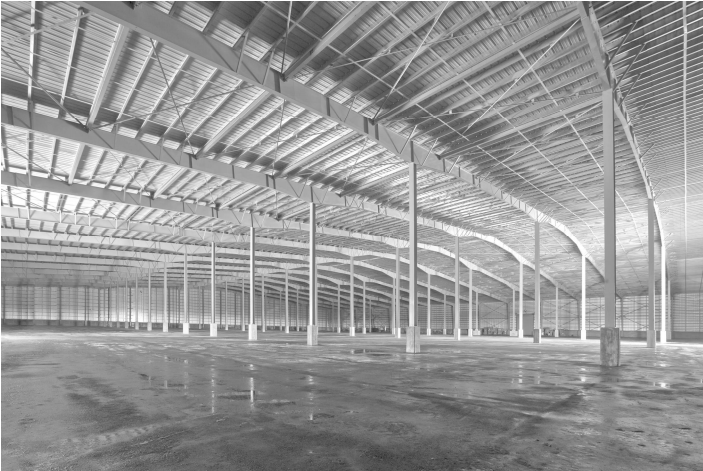
Continuous Beam Frames Sugar Grower's Warehouse-Lemartec Engineering & Construction
