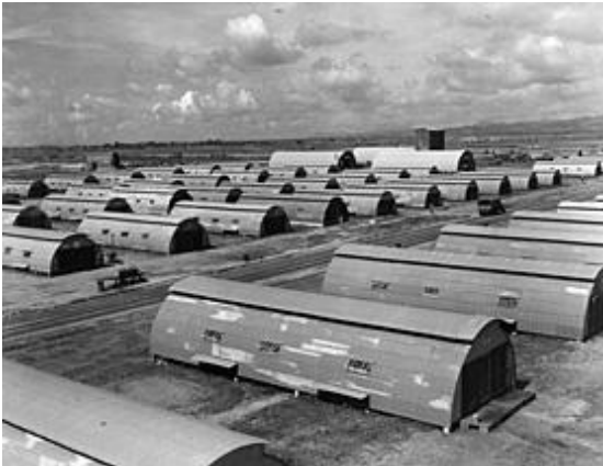
Stran Steel Quonset Huts - 1944
