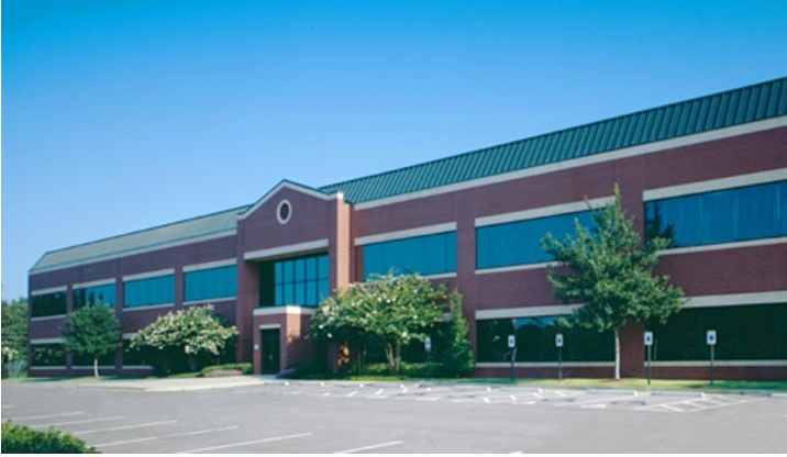
Varco Pruden Buildings Memphis, Tennessee
