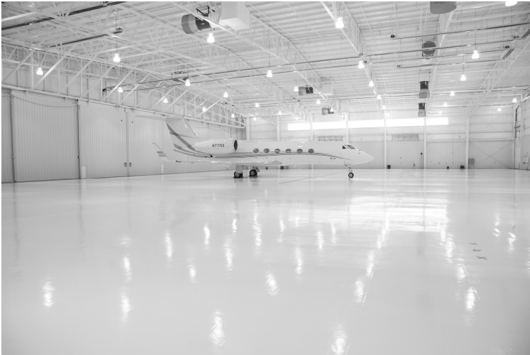
Open Web Frames – General Industries, Charleroi, Pennsylvania Photo courtesy of Don Ivill
